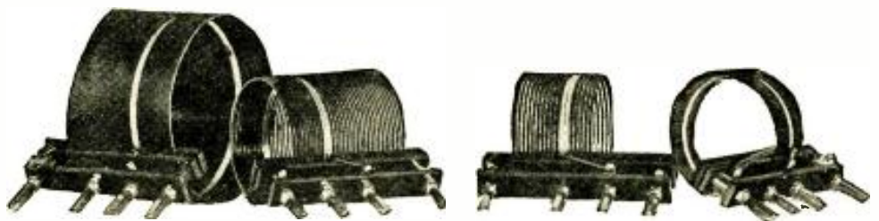
A set of the plug-in coils used in the adapter-receiver, with their standard interchangeable mountings. The space-wound wires are supported on an insulating film.
